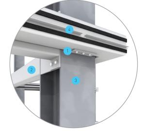
Vertical attachment Qbiss One elements must be made on a horizontal classic steel substructure which is attached to the main structure. The horizontal substructure must be within acceptable tolerances.
