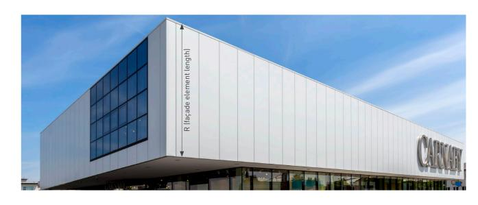
Qbiss One longitudinal corner element completing building envelope.
