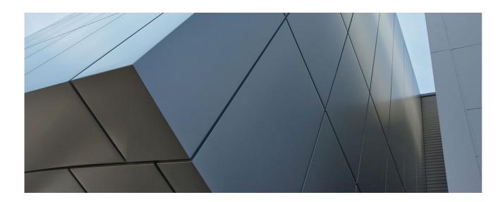
3D corner element was developed in a way that a single Qbiss One corner element is laid horizontally and folded by 45° angle in the transversal direction. This allows façade to pass smoothly into a soffit in one piece. 3D corner elements are possible within horizontal and vertical Qbiss One sys-
